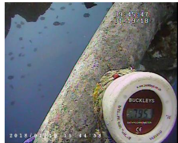
Chain link inspection
